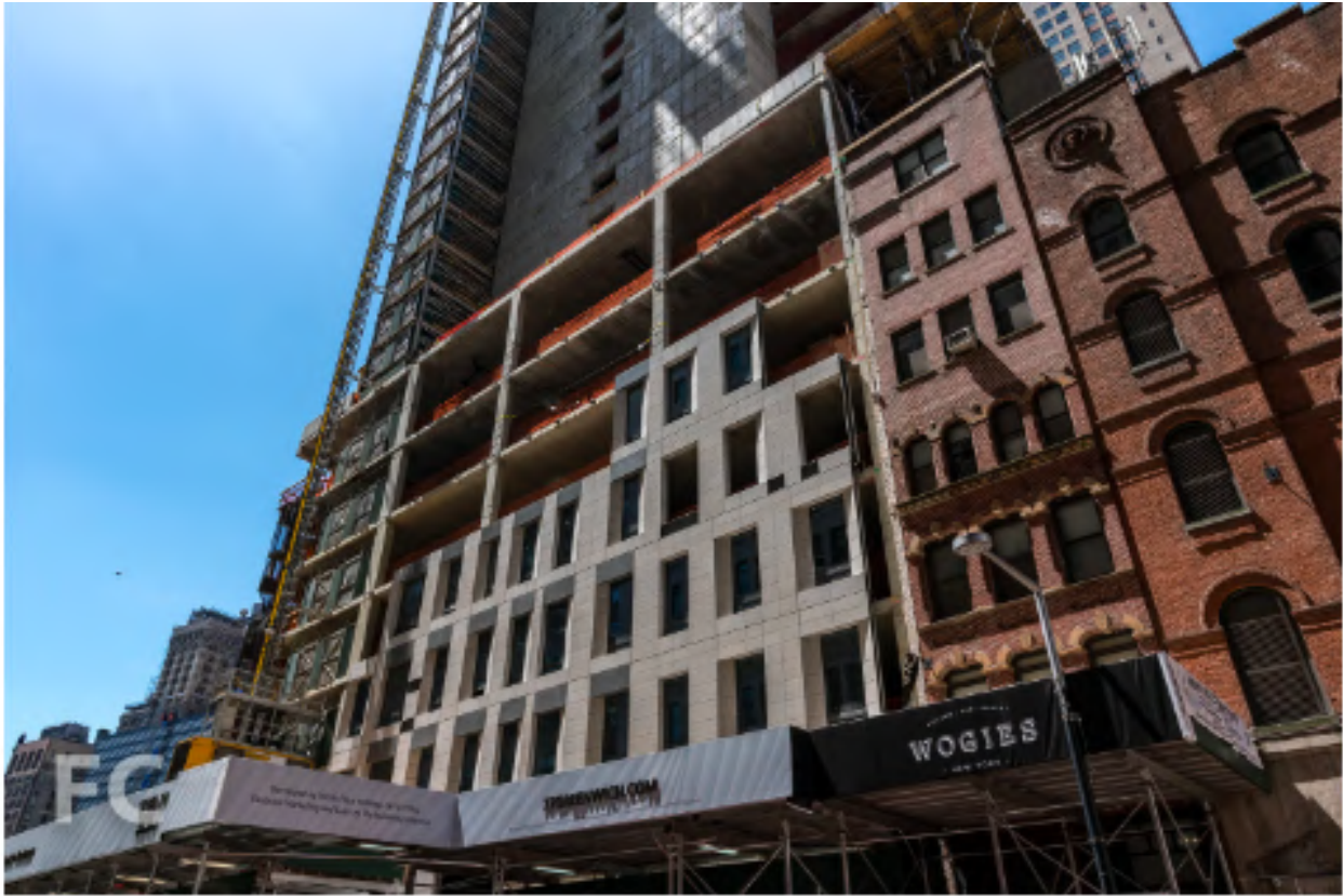
Looking up at the east facade.
