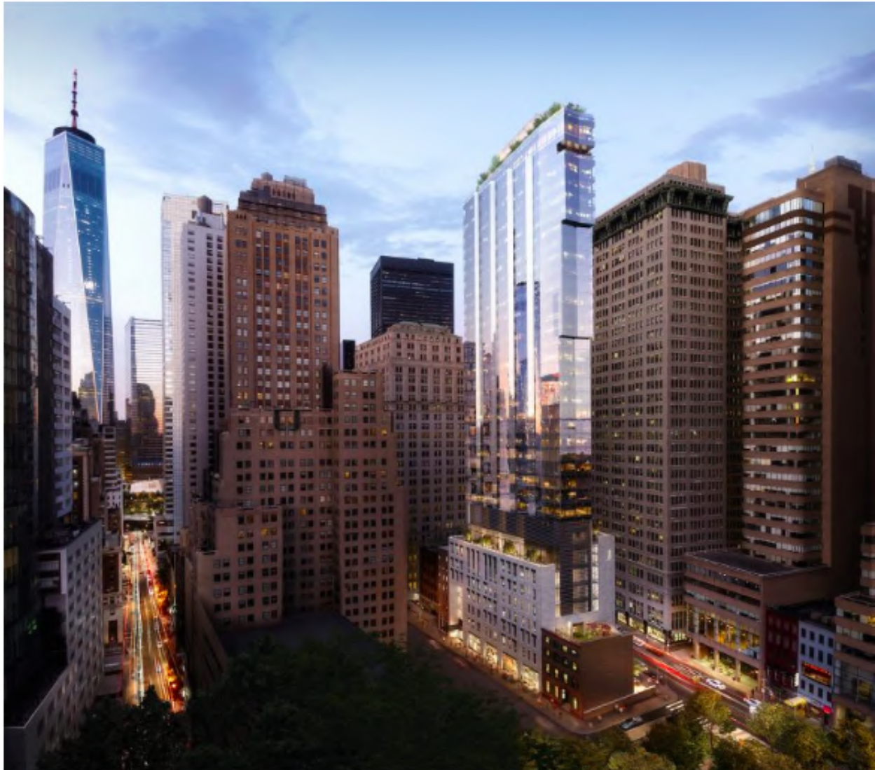
77 Greenwich Street, by Binyan Studios
